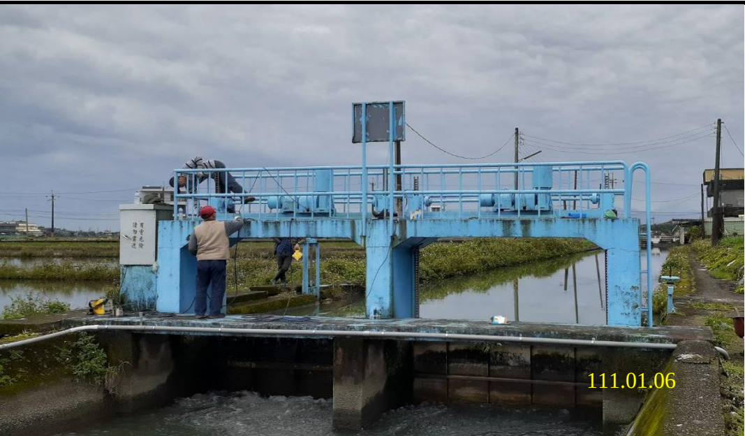
茅埔水門施工前
