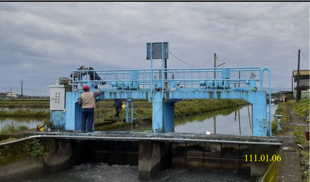
茅埔水門施工前
